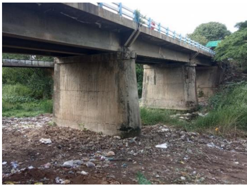
Figure 5. Velanthavalam bridge site
